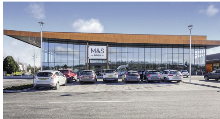
Willowburn Retail Park - Phase 1 due for completion August 2019 to provide 12,000 sq ft M&S Food Hall, Starbucks drive-thru and local artisan country store. Phase 2 will deliver an additional 20,000 sq ft of retail premises
