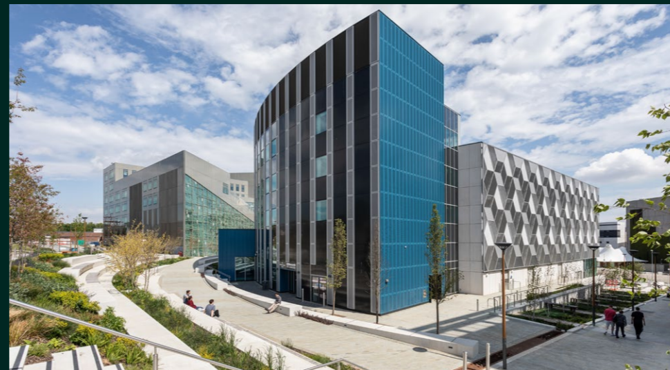
Newcastle University - The Fredrick Douglas Centre
