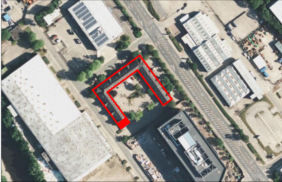
SITE AERIAL VIEW (Building highlighted in red)
