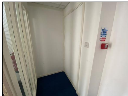
PHOTOGRAPH 11 TYPICAL VIEW OF CENTRAL RISER CUPBOARD AFFORDING VERTICAL ACCESS
