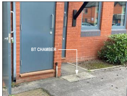
PHOTOGRAPH 8 TYPICAL VIEW OF THE BT CHAMBER ADJACENT TO SERVICES CUPBOARD
