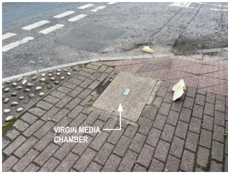
PHOTOGRAPH 4 EXISTING VIRGIN MEDIA CHAMBER IN FOOTWAY ON MAIN AVENUE ADJACENT TO JUNCTION WITH THE WILLOWFORD
