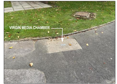
PHOTOGRAPH 6 EXISTING VIRGIN MEDIA CHAMBER IN FOOTWAY ON THE WILLOWFORD ADJACENT TO BUILDING
