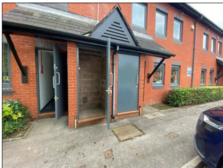
PHOTOGRAPH 7 TYPICAL VIEW OF SERVICE CUPBOARD ACCESSED FROM THE REAR OF BUILDING
