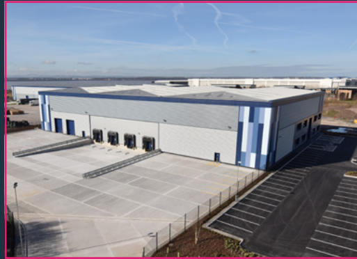
HURRICANE 52 Estuary Business Park, Liverpool
