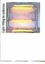
Pendant light - suspended from copper tube frame by electrical contractor
