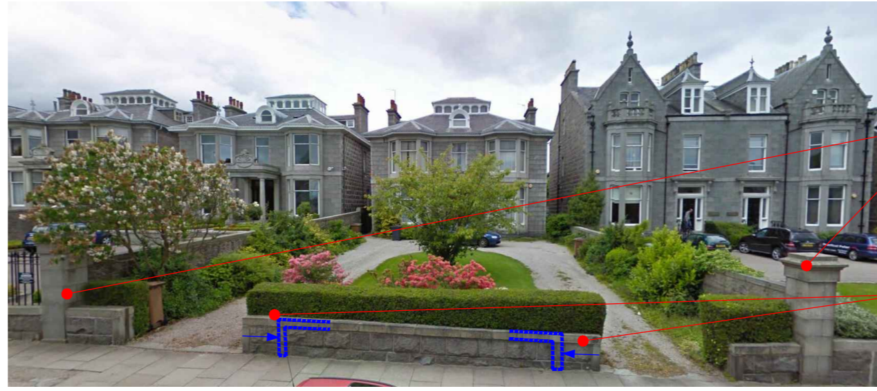
Image of Boundary to Queen's Road South Elevation For scaled drawing please refer to drawing E002
