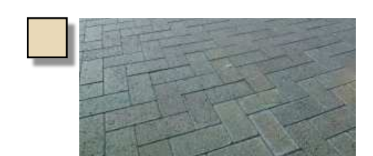
Block Paving Parking Spaces
