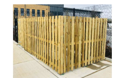
Timber Refuse Area
