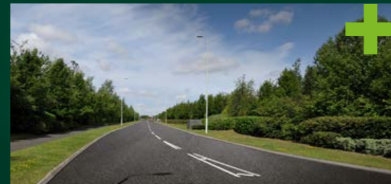
Maintained private roads
