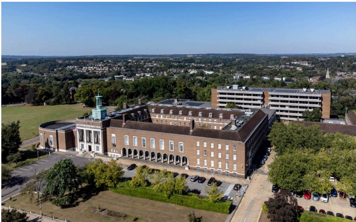
Photograph of the Property looking north
