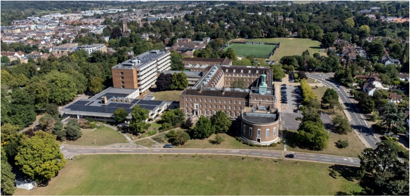
Photograph of the Property looking east
